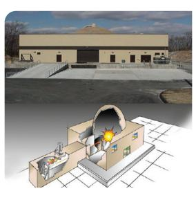
The Davidson Advanced Warhead Development Facility consists of a 40' diameter by 40' tall reinforced concrete dome, lined with armor plate, attached to a 335-ft concrete tunnel for extended warhead to target standoff distances.
